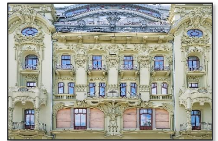
Figure 37. The building of the former Bolshaya Moskovskaya Hotel in Derybasivska Street (fragment), September, 2021
